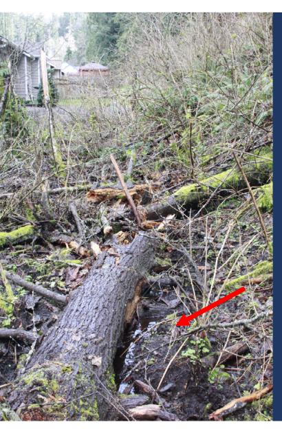
Although the geotechnical reports states that seeps were never observed, I photographed this seep (red arrow) at the toe of the landslide hazard area in the Regatta Estates Tract 992 utility corridor. Homes along 133<sup>rd</sup> Place W are seen to the east.
